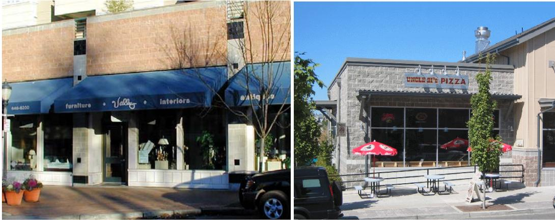
Figure 20.92.200(C). Acceptable use of concrete block on facades. The left image uses smooth gray blocks on the vertical columns and beige split-faced blocks above the awnings. The storefront in the right image uses gray split face (but less than 50 percent of the façade) and some lighter, square, smooth-faced blocks below the storefront windows.
