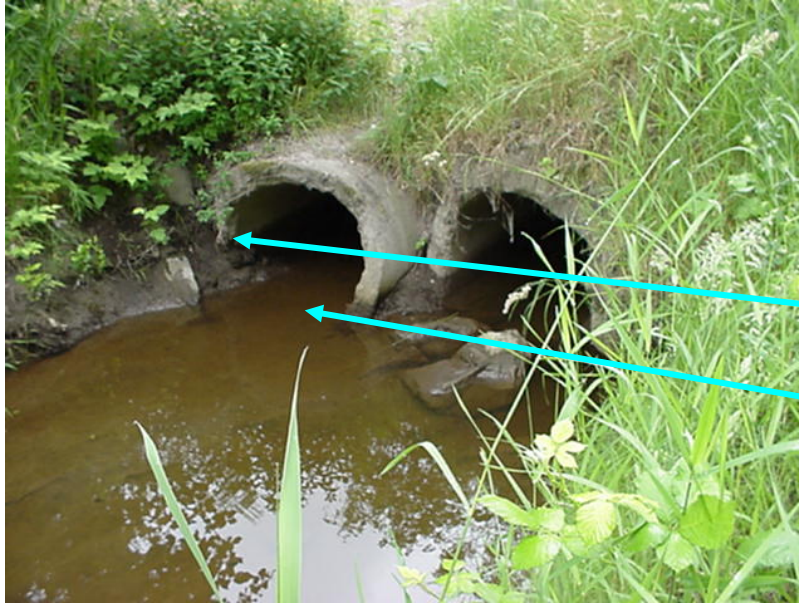
Figure 23: A round culvert with water still present. Measure the distance from the bottom of the culvert, not the present water level. The depth of storage is approximately 5 inches.
