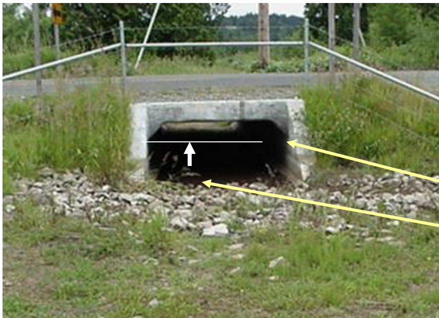
Figure 22: A box culvert that is the outlet of a depression wetland. The live-storage is measured as the distance between the bottom of the culvert and the water marks on the side. The distance is approximately 15 inches.
