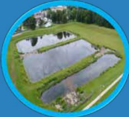
Storm water management
