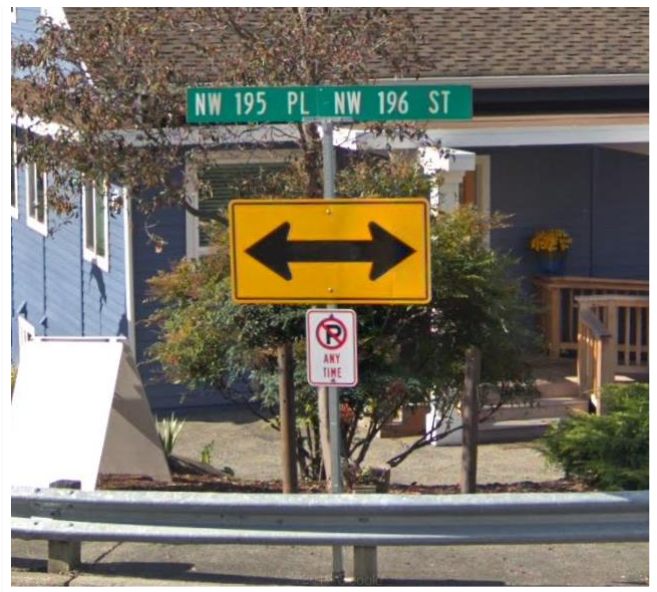
Figure 10. Supplemental no parking sign within intersection
